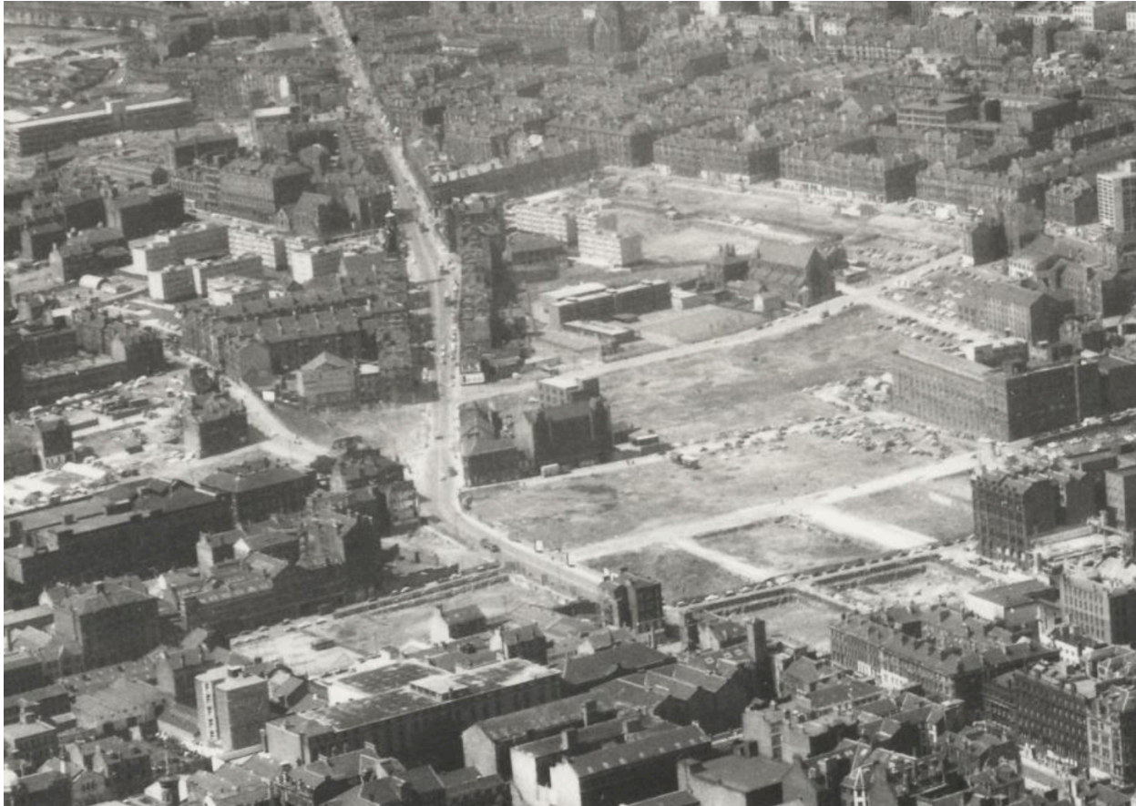
Figure 4.3: 1960s demolition of Victorian tenements (Courtesy of Collective Architecture)
