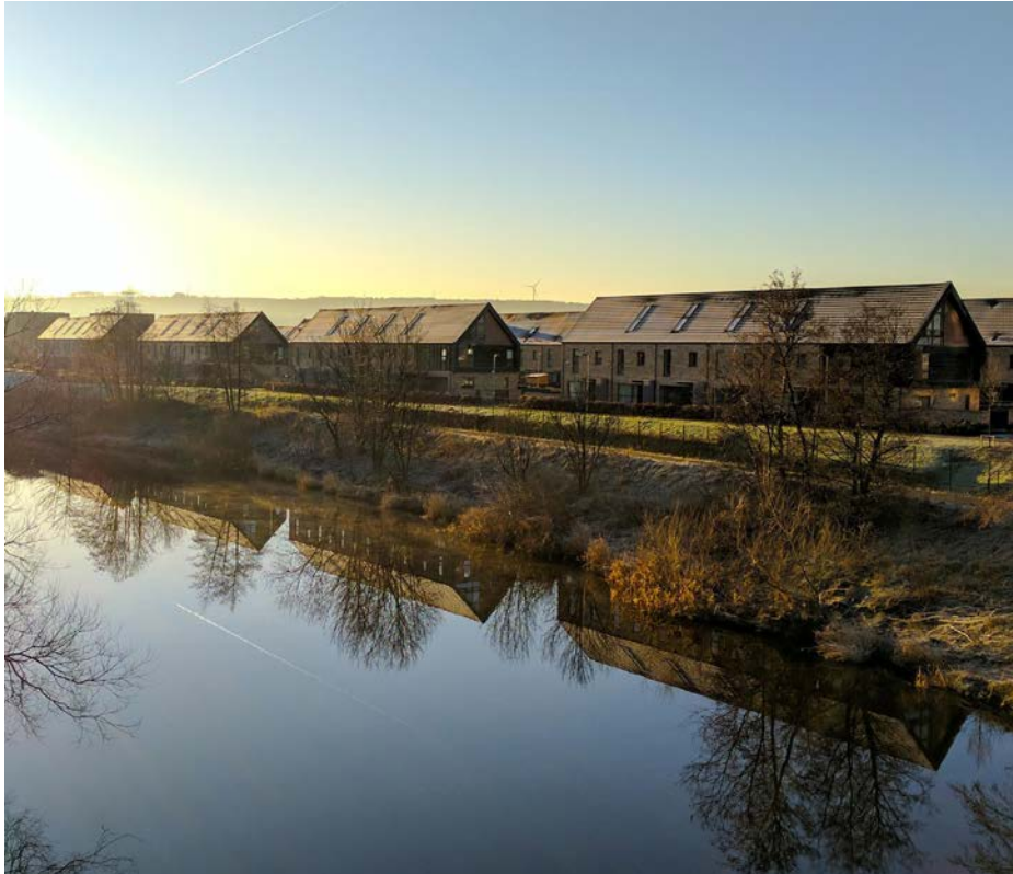
Figure 4.24: Glasgow Commonwealth Games Village, Phase 2 (Courtesy of Stewart Stevenson Architects)
